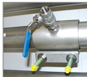
B Spot drilling collars
